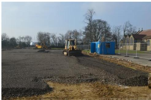
The pitch is being "stoned" ready for the application of the tarmac.
